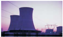
Thermal power station
