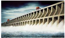
Hydraulic power station
