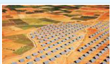
Solar power station
